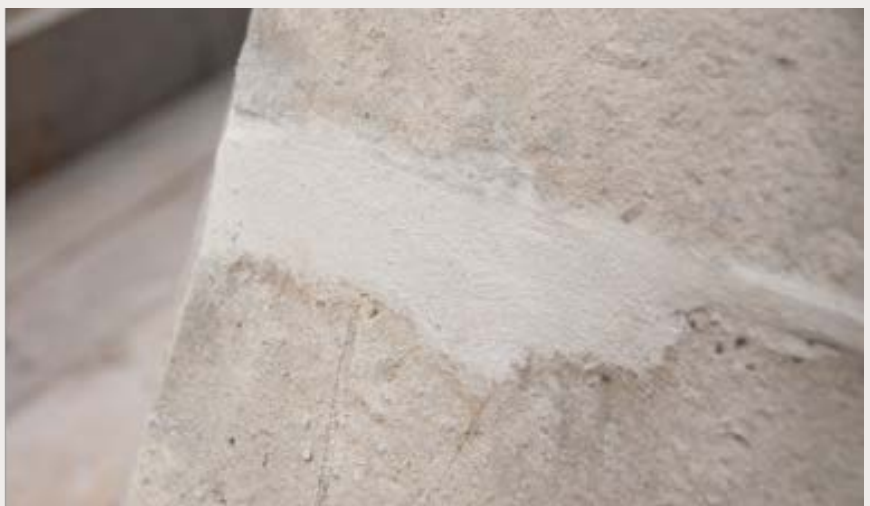
Pinning and re-pointing the Portland stone.
