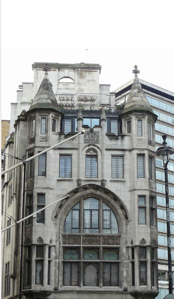
Before restoration work
